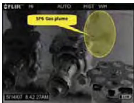
Figure 6. Diaphragm leak.
