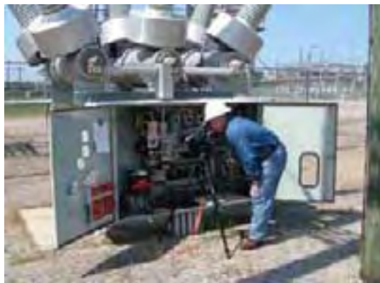
Figure 3. Using the GasFindIR to find and document leaks in an SF 6 compressor cabinet.
