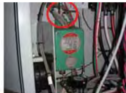
Figure 4. SF 6 leak above pressure switch in compressor cabinet. This cabinet services a 230 KV capacitor bank.
