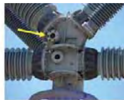
Figure 2. SF6 leak from rupture disk on 500 KV switchgear at 37 feet distance. Note the corrosion around the rupture disk bolts. In the video one can easily detect the leak coming from the bolt in the nine o'clock position.
