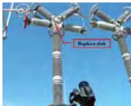
Figure 1. GasFindIR LW viewing rupture disks on 500 KV live switchgear. Inset at right shows the GasFindIR mounted on tripod to exploit high sensitivity mode.
