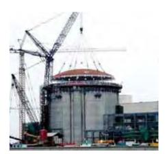
Figure 4: Very-heavy-lift crane and opentop, modular construction at Qinshan Phase III, China
