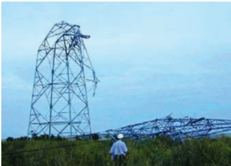
Tower failure due to high winds.
