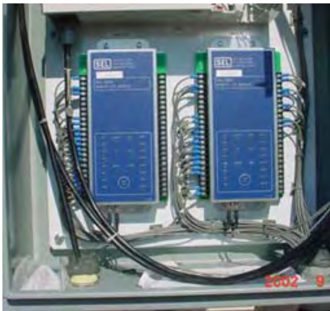
Figure 3. The I/O device on the right provides open and close commands for the MODs. It also provides the 43LR, 52a, and 52b status to the DCS. The I/O device on the left provides inputs into the DCS for the individual power circuit breakers. Note the extra fiber-optic cable, which allowed terminations to be completed in a mobile van and provided additional cable for when the power circuit breaker is replaced.
