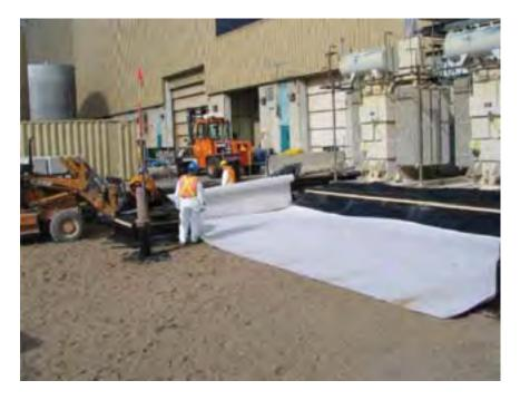
an impervious sheet, typically made of plastic. The plastic will be polypropylene; HDPE; LLPE; PVC, among other types of resins. These sheets of plastic will range in thickness from 0.25
