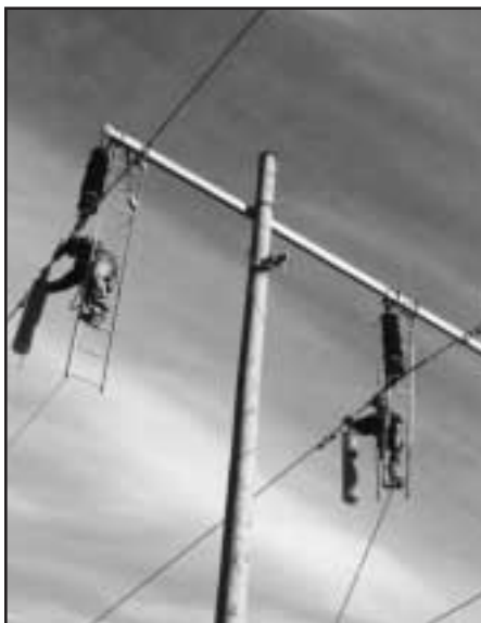
Installing polymer-housed surge arresters on a transmission line – now a safer and simpler task
