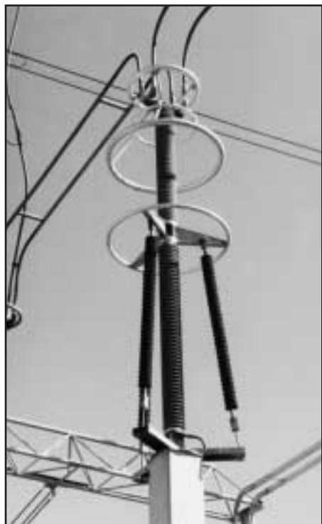
Earthquake-resistant surge arrester with polymer housing
