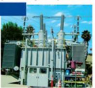
840MVA/500kV Generator Step-UP Transformers for Three Gorges Dam Project, China. 2002
