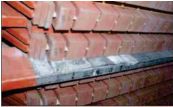
Figure 7: Bar abrasion due to loose windings in the slot of a turbo generator that did not have sufficient sidepacking or a radial follow-up wedging system.
