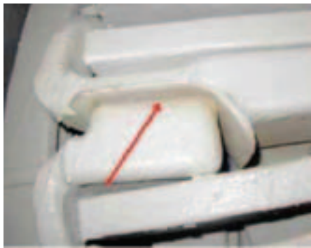
Figure 5: Partial discharges occurring in the inadequate space (here filled with an insulating board) between two phases where the high voltage bars are connected to the circuit ring busses. (Courtesy C. Maughan)
