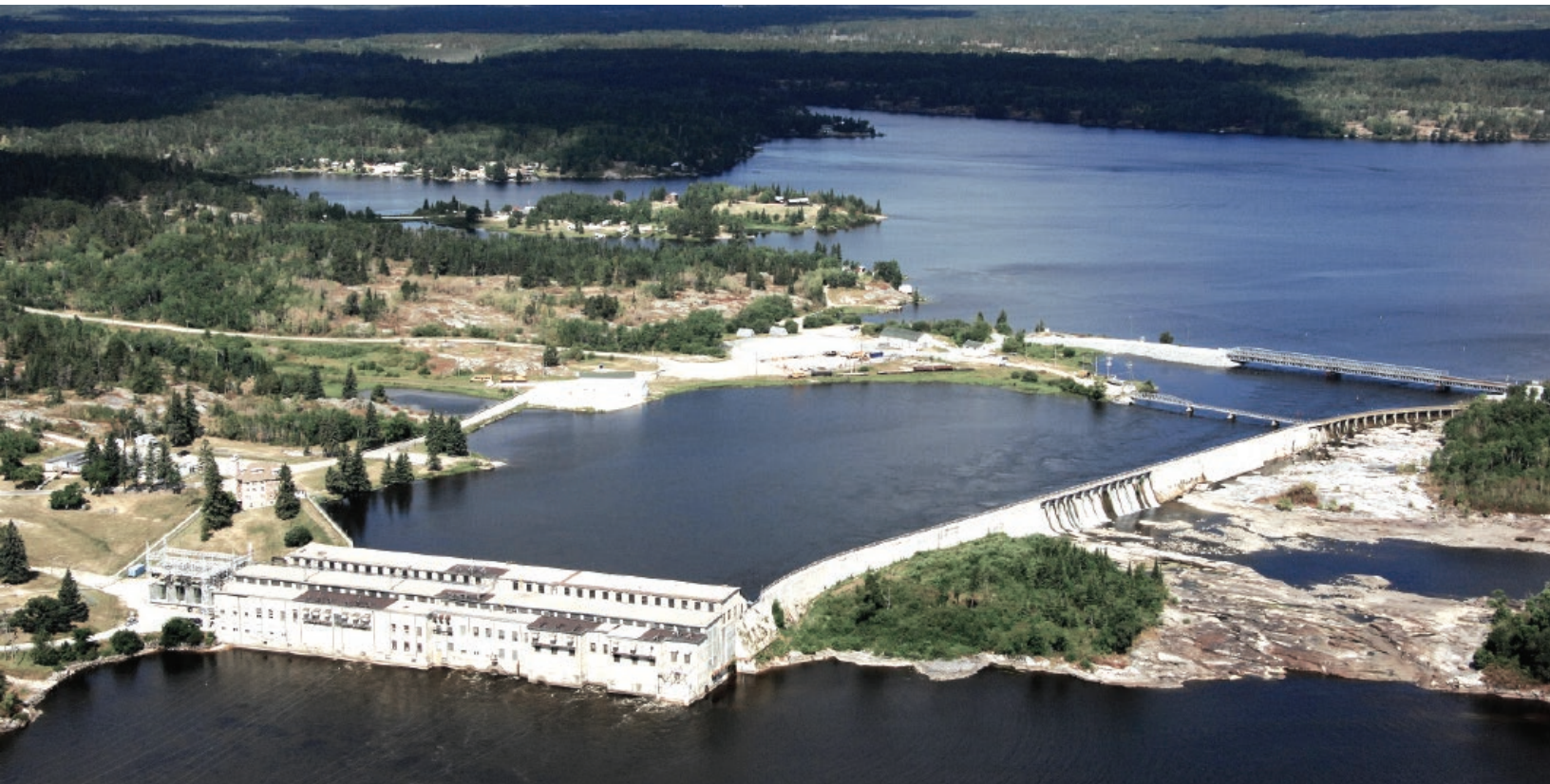
Photo: courtesy of Manitoba Hydro
