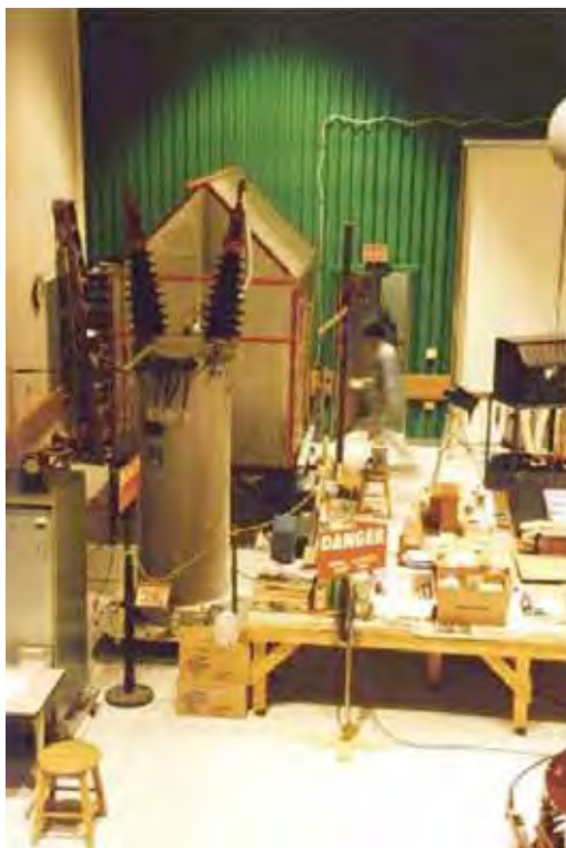
Figure 4. View of the 69 kV fog chamber.
