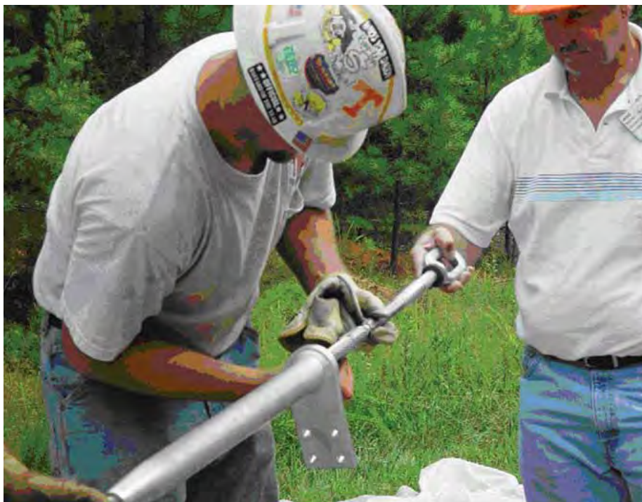
Figure 4: ACCR Larger Outer Sleeve, Which Is Similar to Conventional Conductor Accessories
