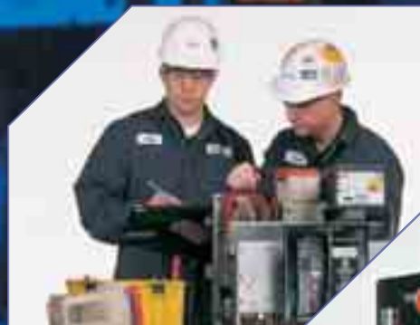
Complete rebuild and NETA certification testing on ITE K1600 ACB.
