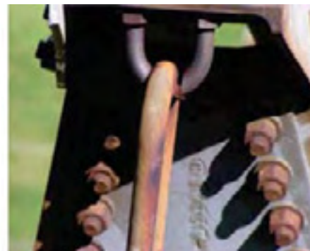
Once an anomaly is detected, a closer view can be established.
