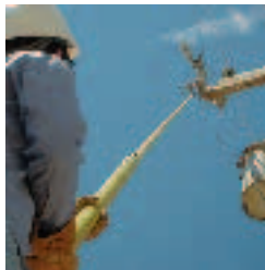
Maintain proper distance when re-fusing.
