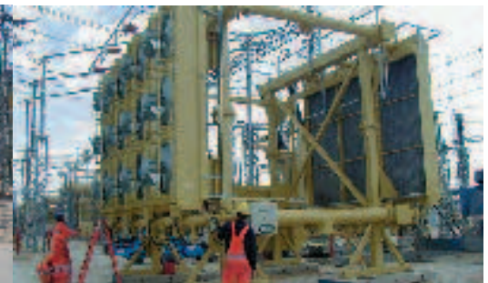
After installation: Notice improved airflow and access for maintenance.
