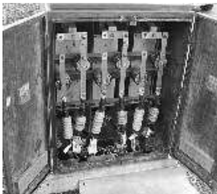
Figure 4: Cable segments ready for injection
