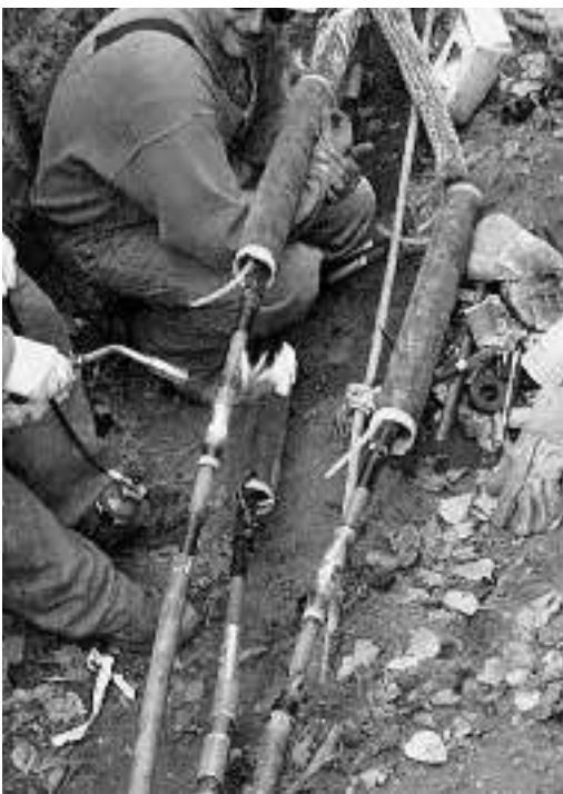
Figure 6: Saskatoon Linemen replacing splices.
