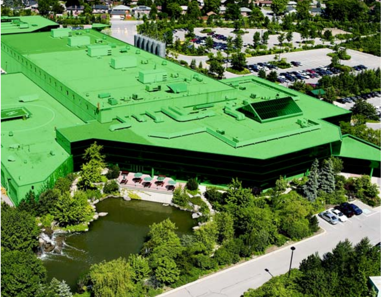
Husky Injection Molding Systems, Bolton, Ontario
