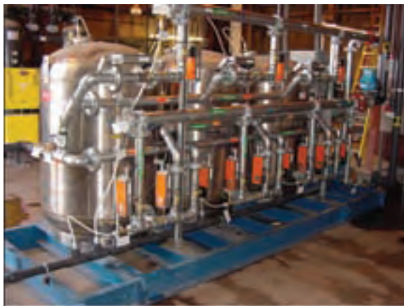
Centrifugal filtration sand filter systems are often the best solution to processed water demands.
